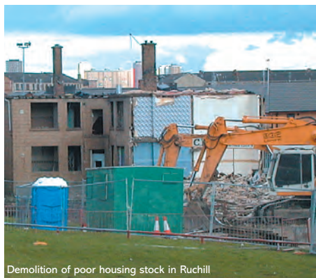
Demolition of poor housing stock in Ruchill
